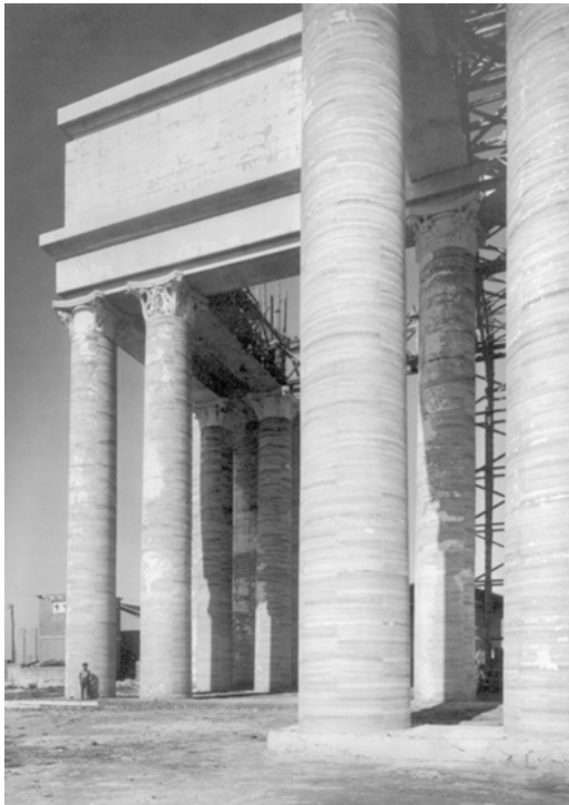
Figure 1: Angiolo Mazzoni, Termini Station, Rome, 1941, mockup of the frontal portico realized in Acque Albule near Tivoli
